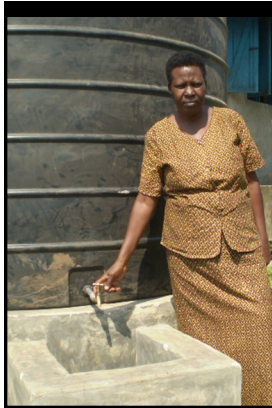
AYA Regional Director Mary at one of the USAID-funded clean water projects in Fort Portal, Uganda
